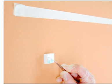
PIC 5-5: Remove the protective cover.
