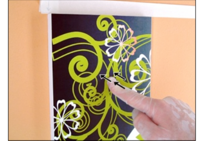
PIC 5-8: Use brief, light presses to stick entire block surface to panel.
