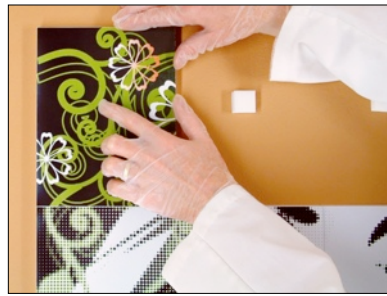
PIC 9-3: Align panel and apply gentle pressure to close gap.
