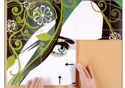
PIC 7-5: Align edges and apply gentle pressure to close gap.
