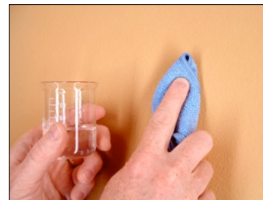
PIC 2-3: Cleaning the wall thoroughly is best.
