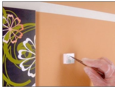
PIC 6-4: Remove the protective cover.
