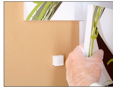
PIC 8-7: Pressure by the block will cleanly separate the panel.
